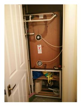
Elson tanks are a relatively old type of hot water storage unit and are quite rare as many have been replaced. However, the convention states that the insulation thickness should be recorded where possible and entered as factory applied insulation. If you are unable to measure the insulation thickness, then "no access" should be recorded. There is also no assumption for a cylinder thermostat so you should check for its presence.
