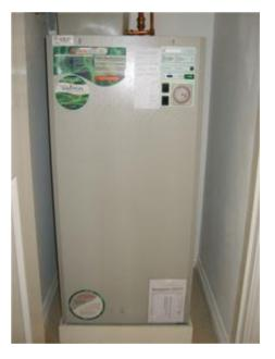
The above are all unvented pressurised steel or plastic encased hot-water storage units. Despite their differing appearance and volume, the insulation is recorded in the same way for each as 50mm factory-applied foam. Please also note that it is also assumed that there is a cylinder thermostat present.
