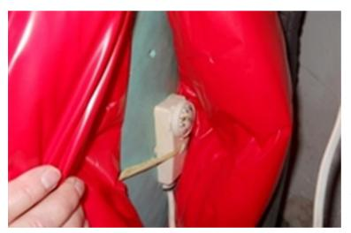
There may be some cases where you find a cylinder that has both spray foam and jacket insulation. The convention has been recently updated to explain how this is recorded. It explains that you should record the thickness of the spray foam, plus 1/3 of the depth of the jacket.
