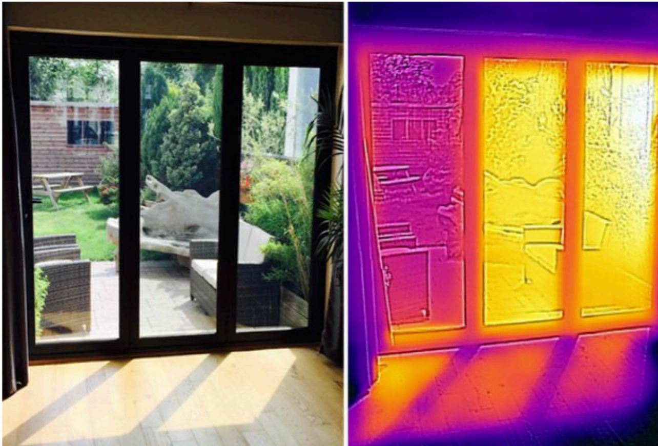
One glazed door covered in solar shading film
