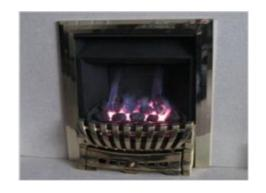
Decorative fuel effect gas fires are the least efficient type of gas fire at 20% efficient. The identification of this fire is the chimney - it will be fully open with a diameter more than 200mm. Therefore, the chimney is included in the open fireplace count. The unit itself sits on the grate (look for evidence of a gas pipe) and the heat is allowed to escape up the chimney.
