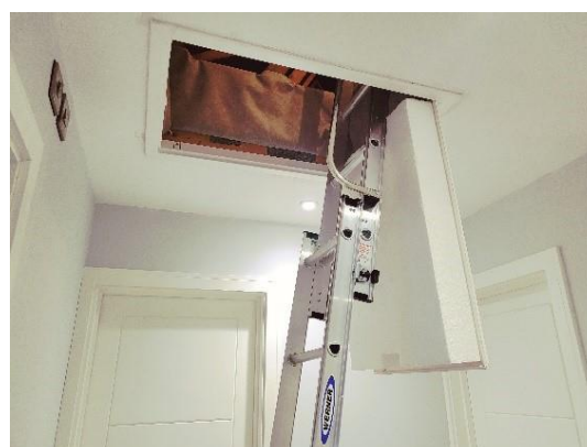
Figure 2 Proprietary hatch insulated with polystyrene board and draught proofed
