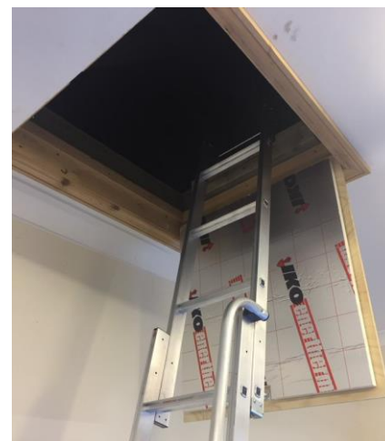
Figure 1 Loft hatch insulated with foil backed PIR Board
