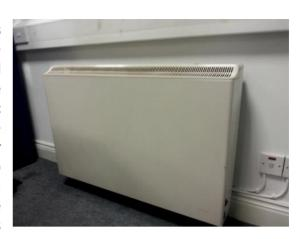
Another indicator is separate controls for the storage heater and the direct acting heater. In the examples on the right, the storage heater controls are on the top of the unit and the direct acting controls are on the side of the unit. They are typically located near the front of the unit as this is where the direct acting heater is situated.
