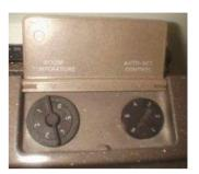
Automatic charge control is quite rare and can be achieved using internal thermostat(s) or an external temperature sensor to control the extent of charging of the heaters. Availability of electricity to the heaters may be controlled by the electricity supplier based on daily weather predictions when used in conjunction with a 24-hour tariff; this should be treated as automatic charge control.
